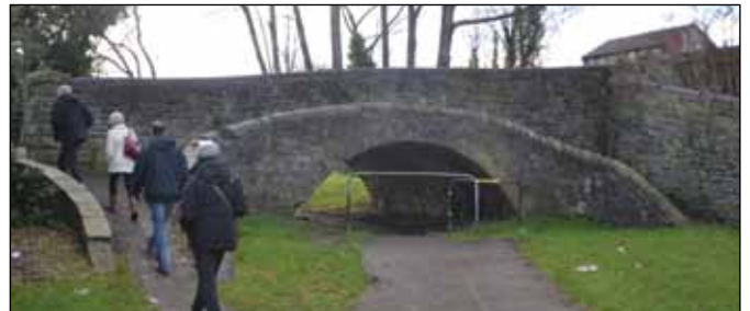
Figure 11: Morfydd Street bridge (Grade II)
