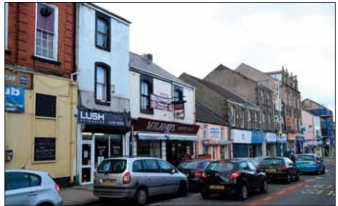
Figure 37: Variation in upper storeys of buildings along Woodfield Street
