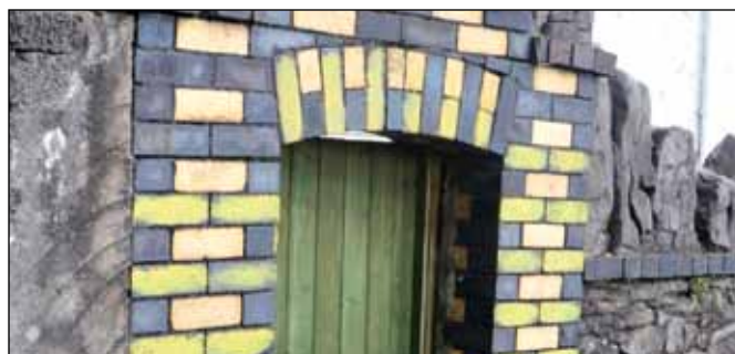
Figure 34: Use of copper slag in local walling highlights the industrial past
